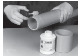
Apply solvent cement to the outside of the pipe
