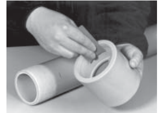
Abrade pipe and socket
