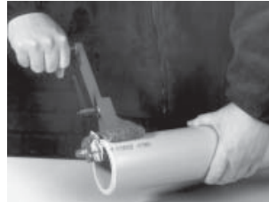
Deburr/chamfer
