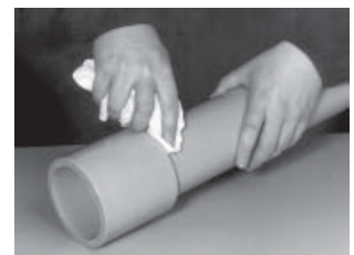
Wipe off excess solvent cement
