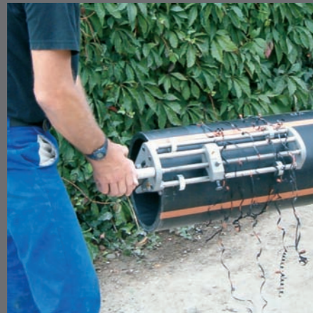
Optimum removal of the oxidic layer: a FRIATOOLS scraper tool being used.
